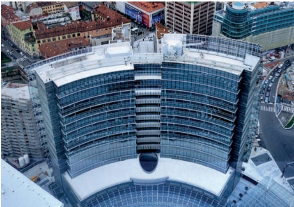
C30.1 EXTERIOR PELLI COMPLEX
