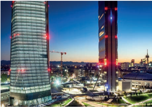
C18.1 TOWERS OVERVIEW
