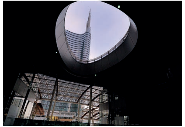
C28.2 FROM PELLI TOWER BASEMENT
